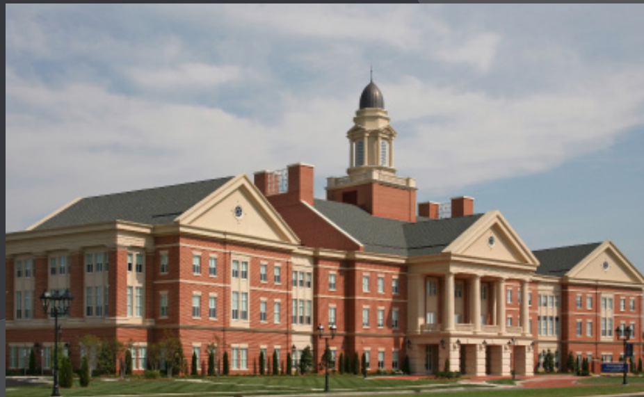
KANNAPOLIS MUNICIPAL CENTER & POLICE HQ
